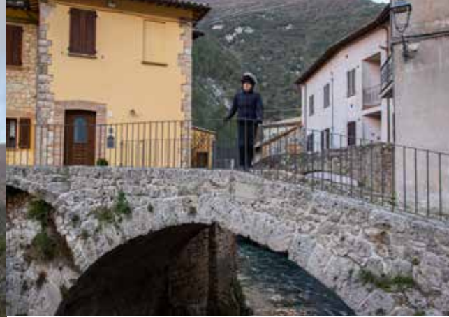
Pioraco, Marmone Bridge
